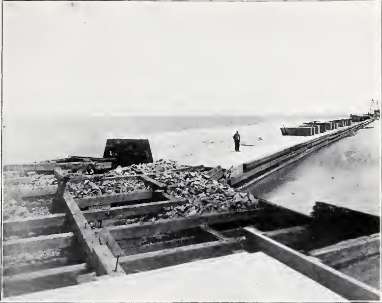
CLEVELAND BREAKWATER. SHOWING ORIGINAL AND MODIFIED CONSTRUCTION The Original Construction was Cribwork—the Modified Construction was Concrete Superstructure
